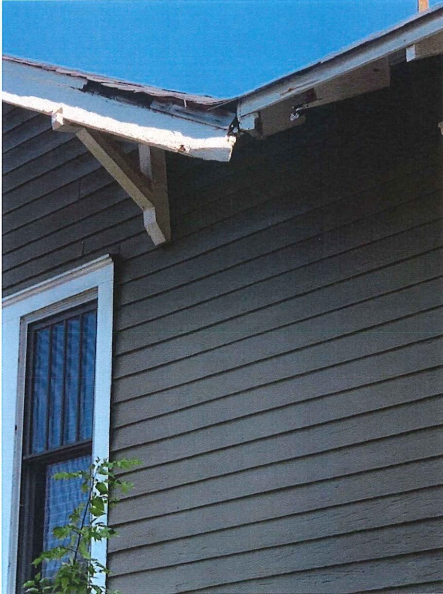
Replacing all rotten fascia boards around the house using the same type of board that is currently used on the house.
