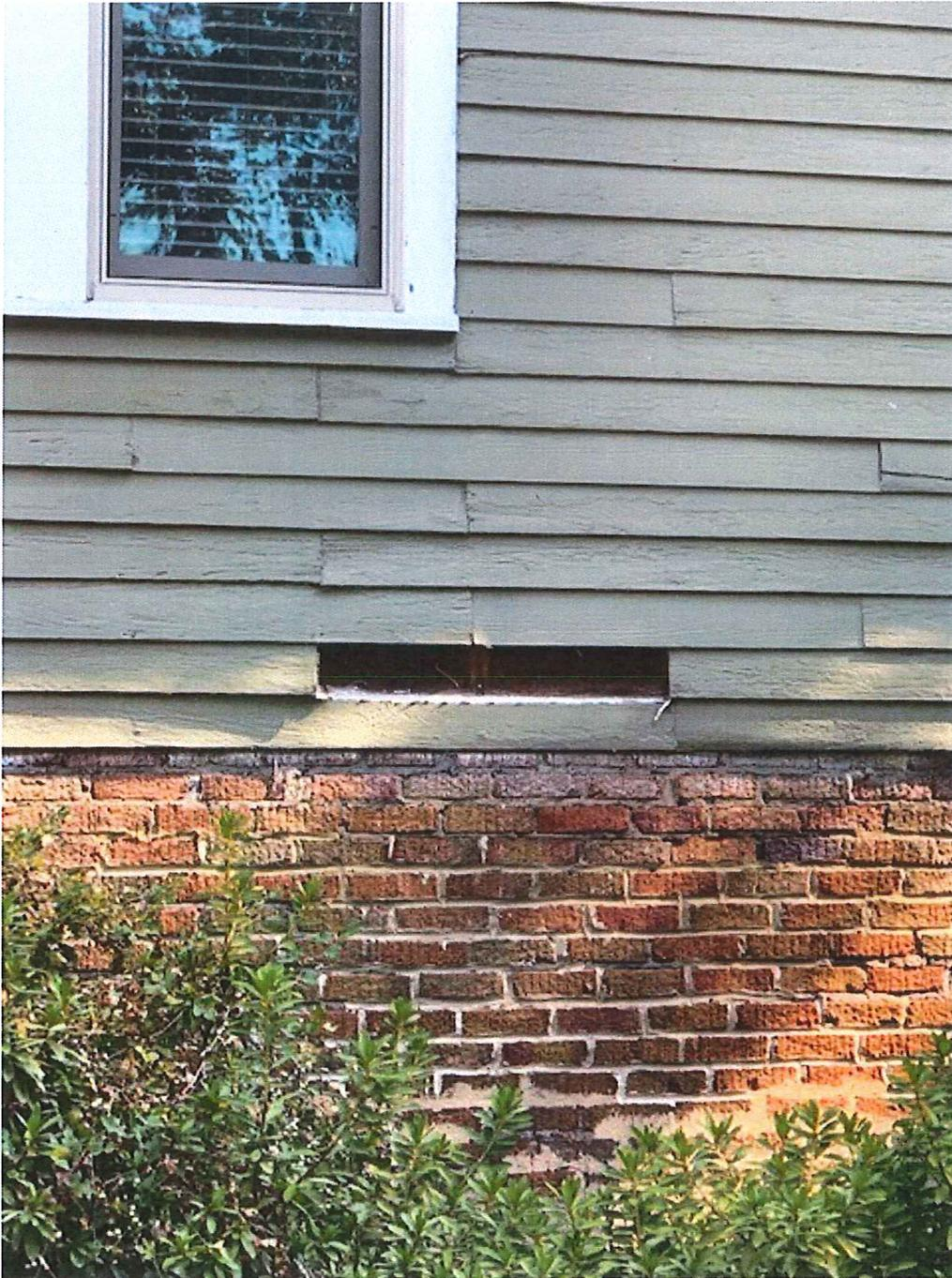
Replace rotten, warped or missing boards with same type of existing boards.
